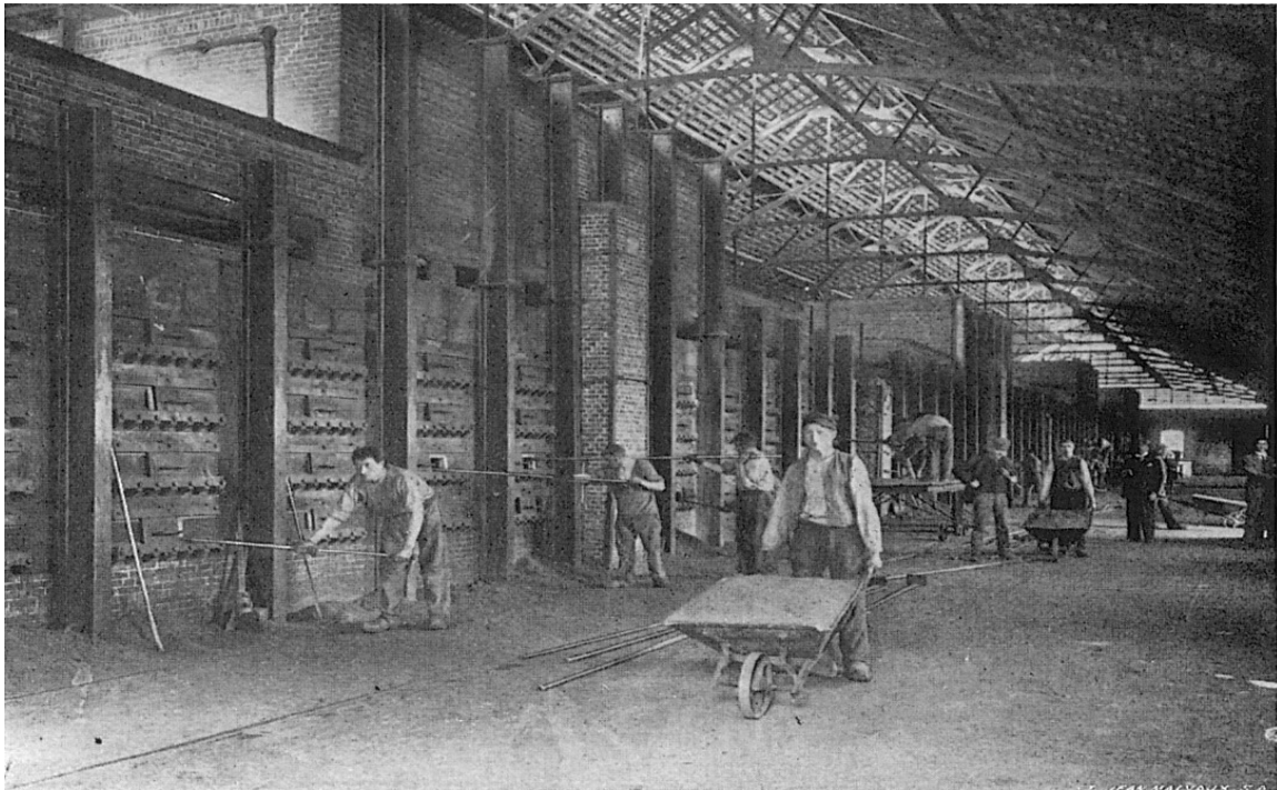
Hall 1 starts with 20 reverberation furnaces for blende with each 2 or more roasting floors.
